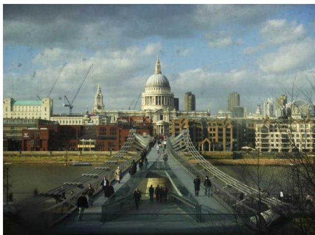
2-rasm. "London Millennium Footbridge" ko'prigining umumiy ko'rinishi.
