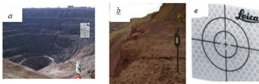
Fig. 2: a, b - the location of the working benchmarks on the ledges; B - view of the luminous observation mark.
